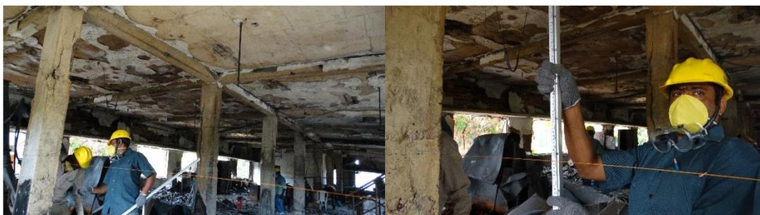
Fig.6 : typical view of levelling and the measurement of sectional deflection
