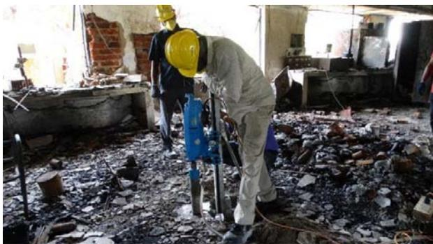
Fig.5 : Concrete Core Extraction on Slab in Progress
