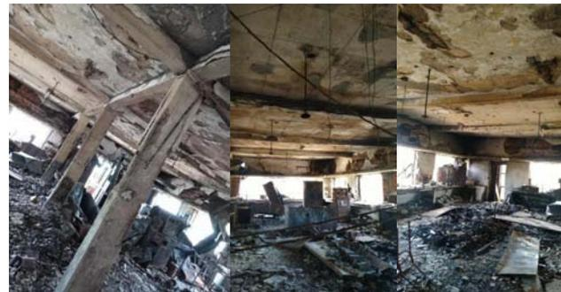
Fig.2 : Typical view of fire damage in first floor of fire affected Building
