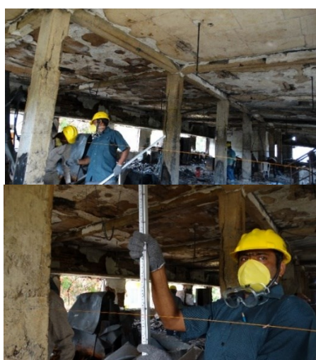
Fig.6 typical view of levelling and the measurement of sectional deflection
