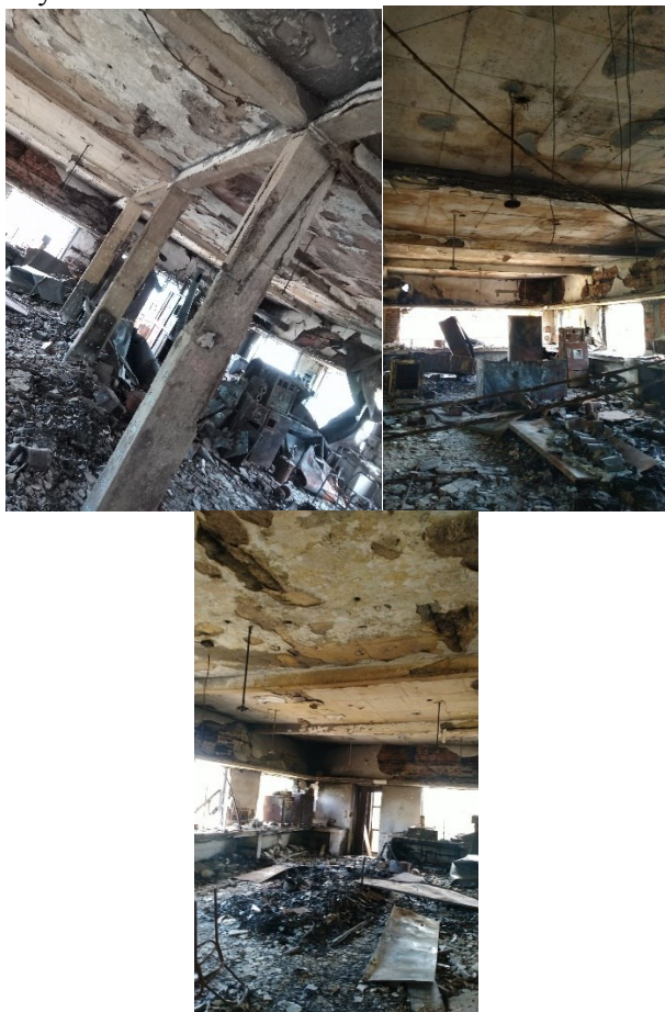
Fig.2 Typical view of fire damage in first floor of fire affected Building
