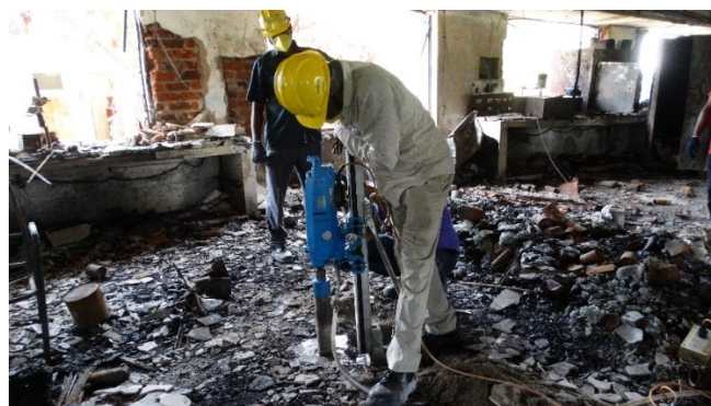
Fig.5 Concrete Core Extraction on Slab in Progress
